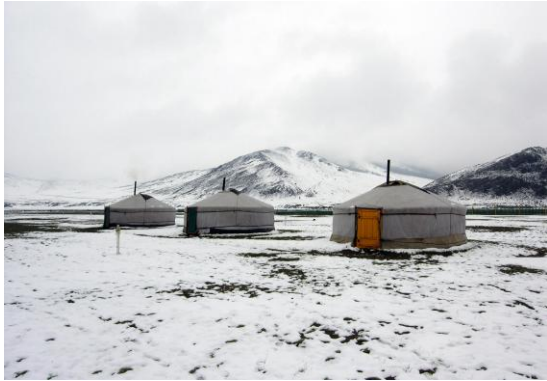
Yurt Circular tent with a timber frame and insulated fabric walls; stable and weather-resistant.
